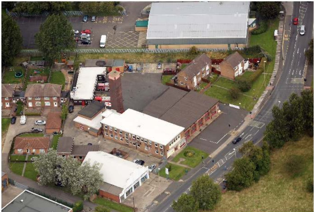
Hebburn Community Fire Station
